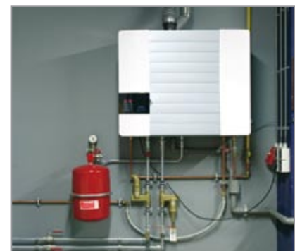
Individual deaerator and dirt separator in a domestic heating system
